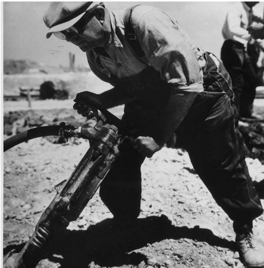
"Photographic Section-Information Service-Works Progress Administration-Washington, D.C. A man at work with Jack-hammer." 1935. Franklin D. Roosevelt Presidential Library & Museum. Photograph: 53227(1957). http://www.fdrlibrary.marist.edu
